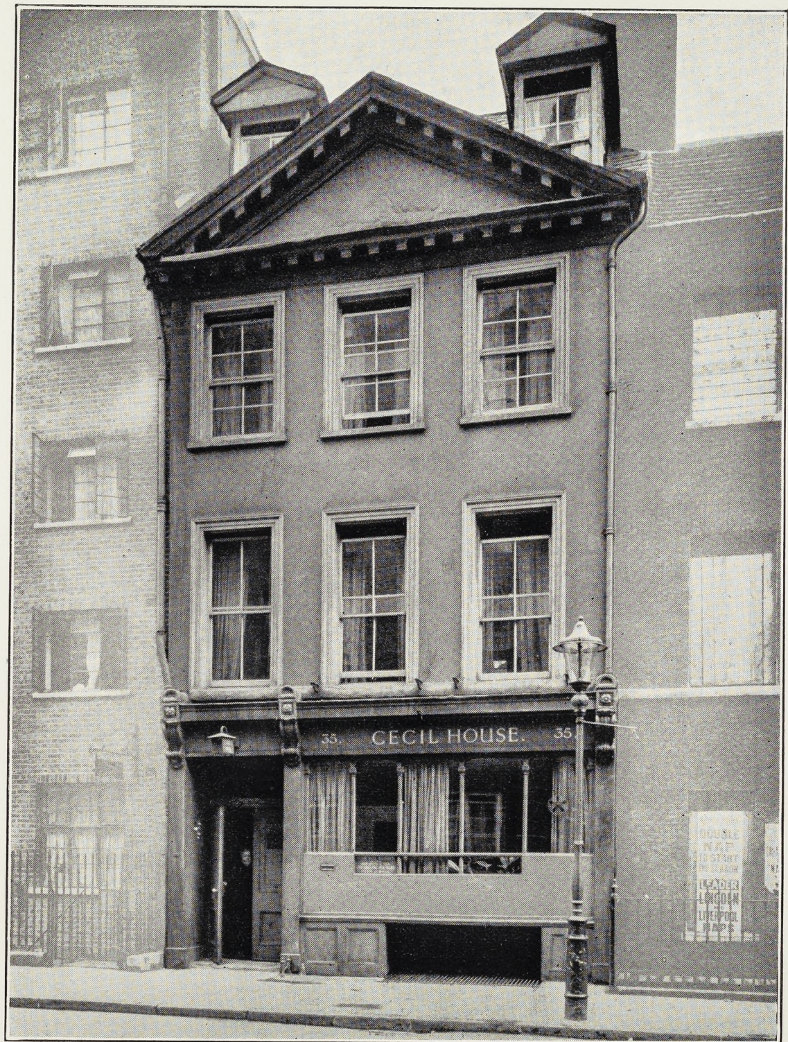
OUR FIRST LITTLE HOUSE—NOW BEING REBUILT ON ENLARGED SITE
