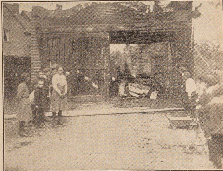
Ruins of Motor Garage Handsworth, Birmingham.
