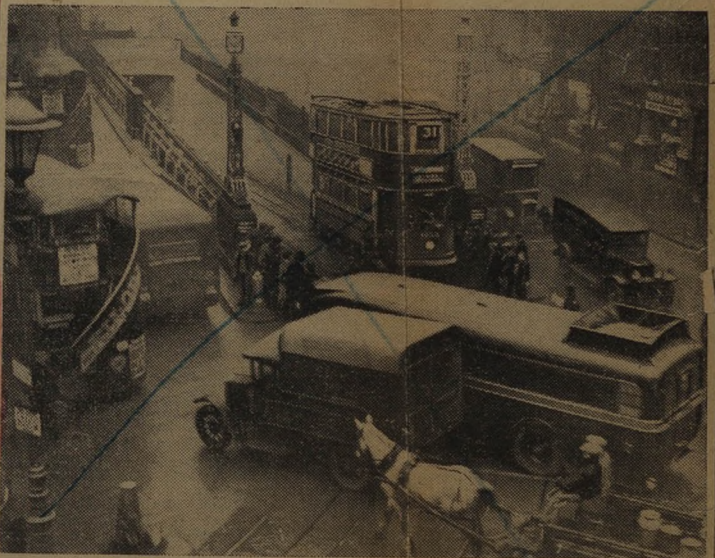
Double-decker tramcars can now come up to Southampton-row from the Embankment by way of the enlarged Kingsway tunnel, but there is really not much room for them when they do. Even without them the problem of keeping traffic moving at a reasonable speed at the point where they emerge is a considerable one.
