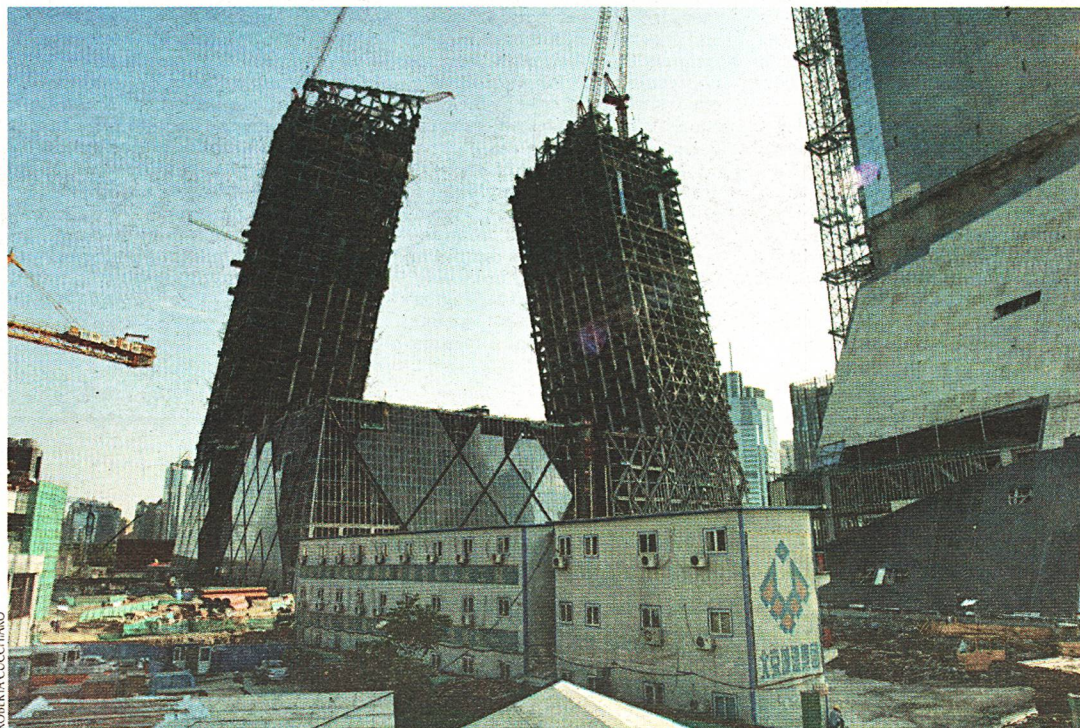
OMA's China Central Television Headquarters in Beijing, under construction in 2007
