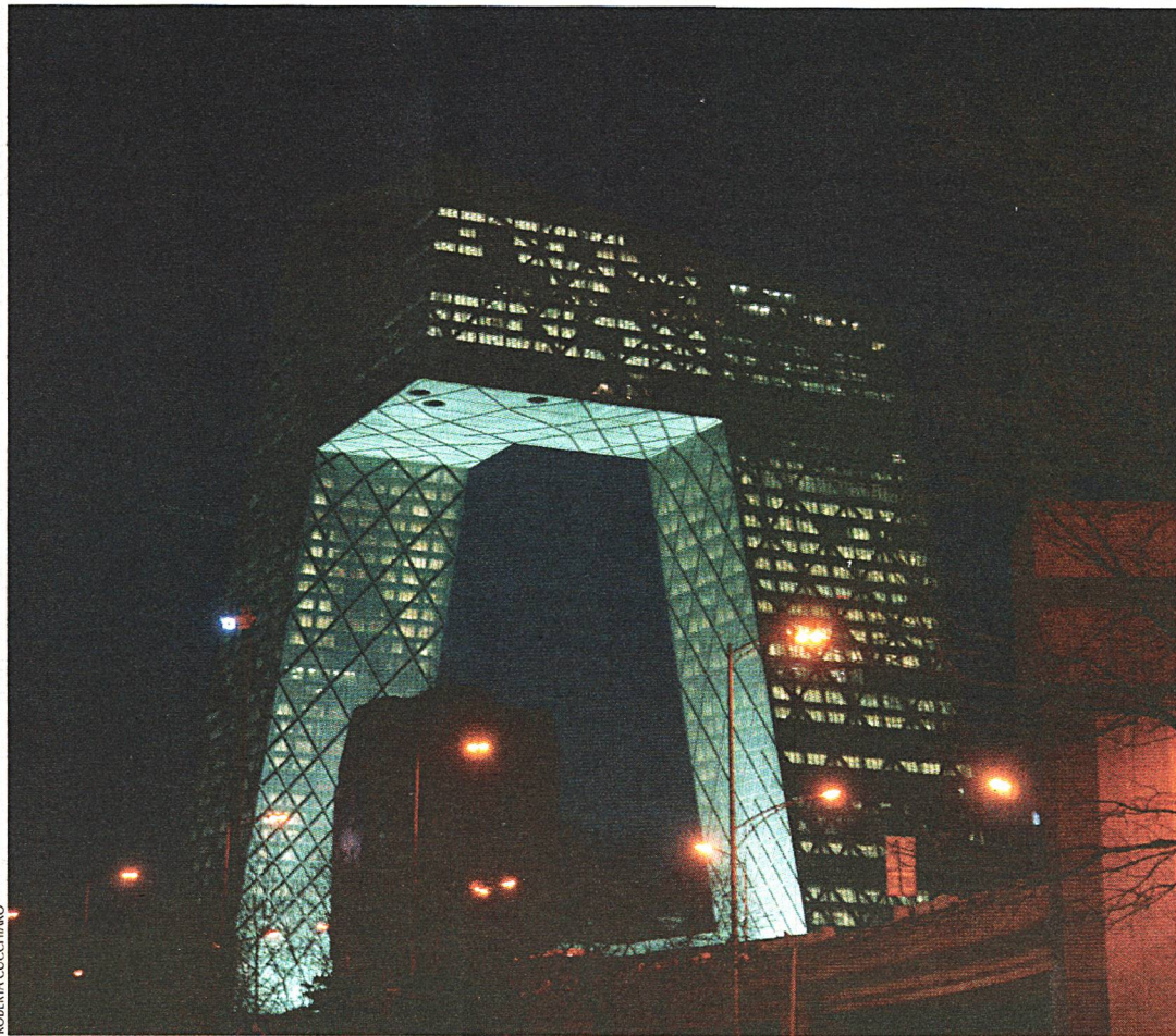
OMA's China Central Television Headquarters in Beijing, by night
