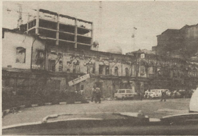
The gutted Bristol Building, The Fort Colombo, which had been full of Tamil businesses. This photograph was taken in secret from a car window.
