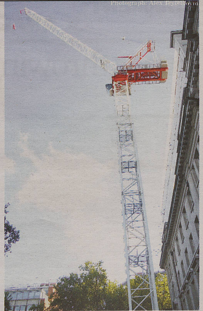
The New Academic Building is still under construction
