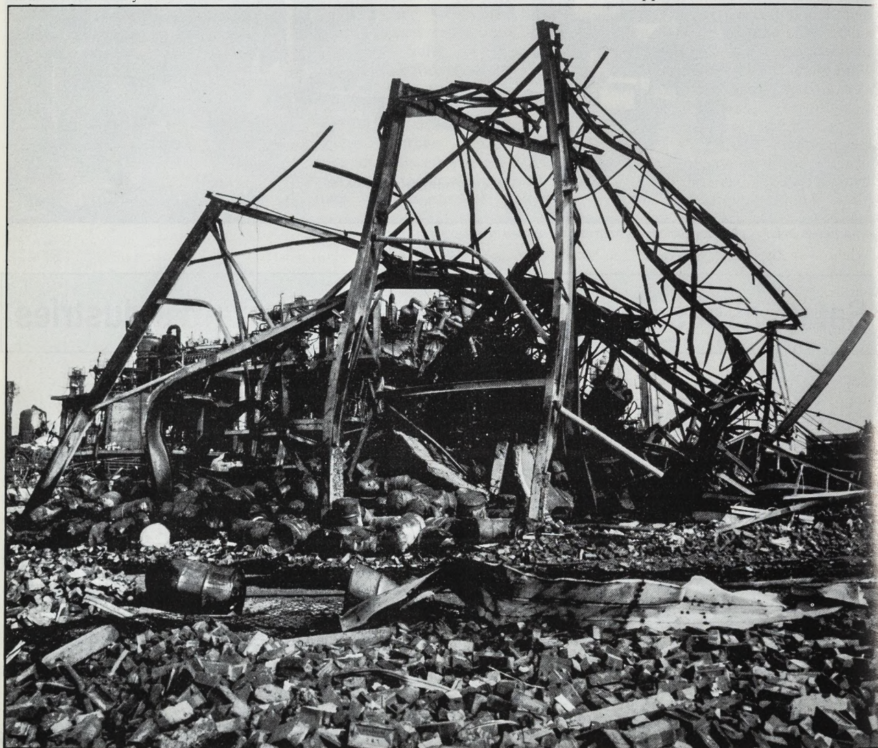
Many parts of onshore installations are certified in one way or another.
