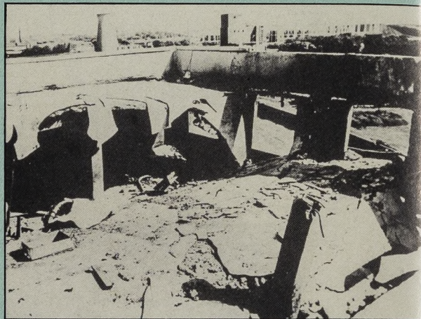
Devastation: The aftermath of a dust explosion at the Spillers flour mill at Bow in 1966. Top: interior. Bottom: exterior.
