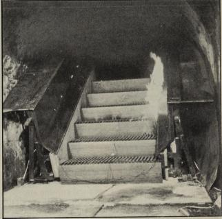
Section of escalator on fire — after four minutes.
