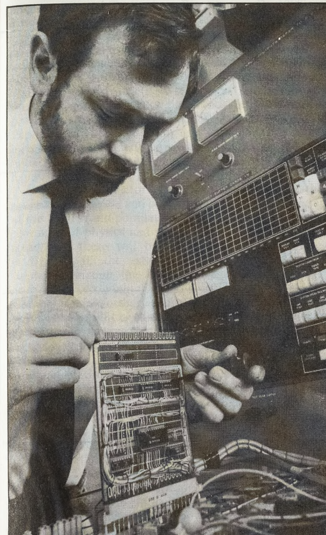
Telephone System circuit board
