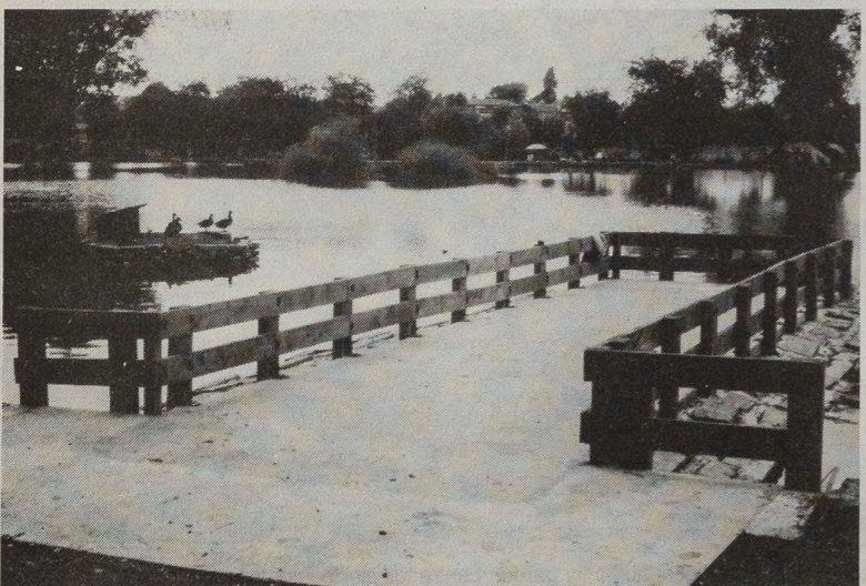
The finished pier.
