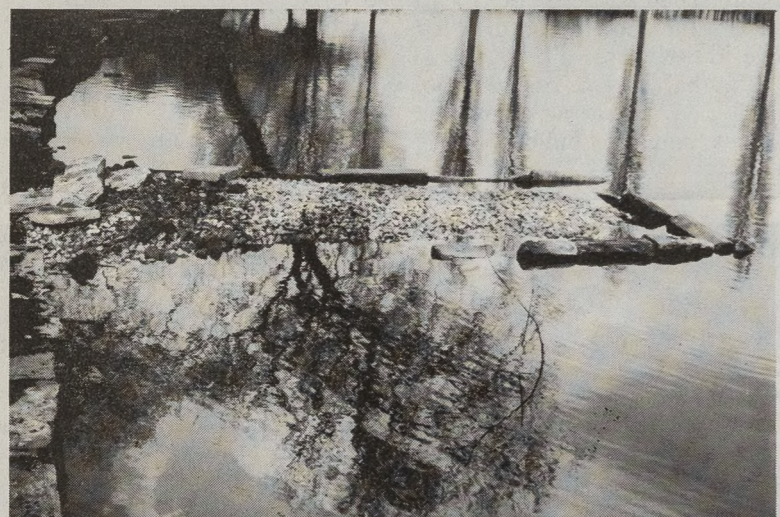
Foundation of pier laid using large sandstone blocks and hardcore binding.
