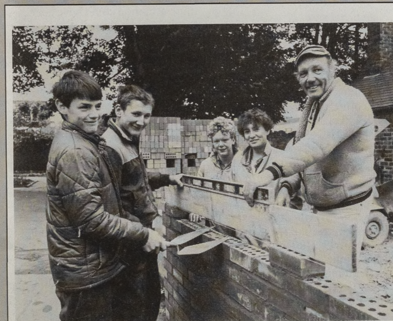
Learning construction techniques on the garden site.
