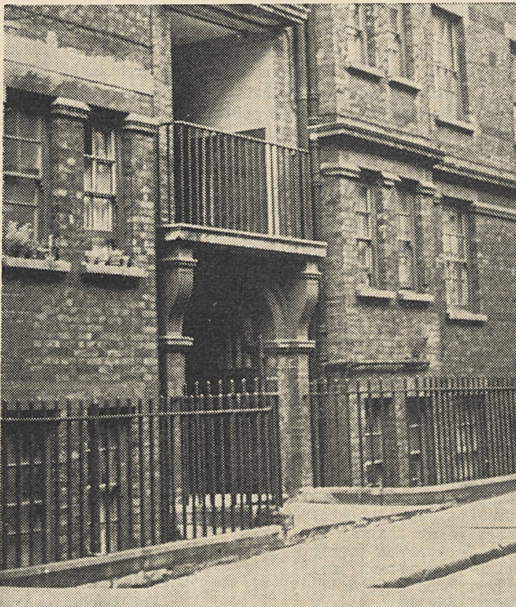
Looks rather like Coronation Street. Tough and dirty but reasonable. Just through that archway you come to this unknown community. Conditions—rock bottom.
