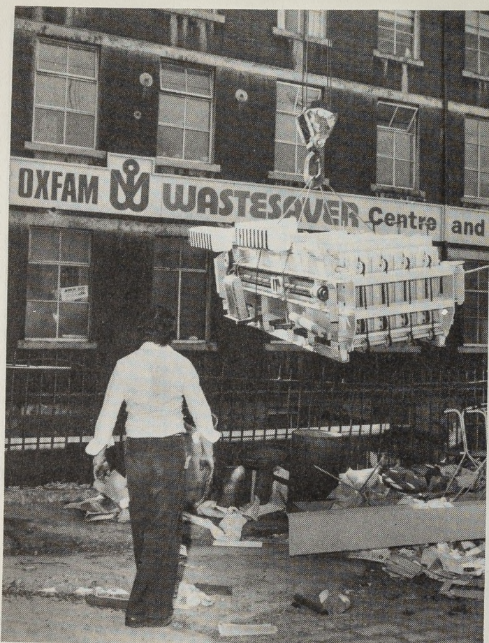
A new baler being craned into the Wastesaver Centre.
